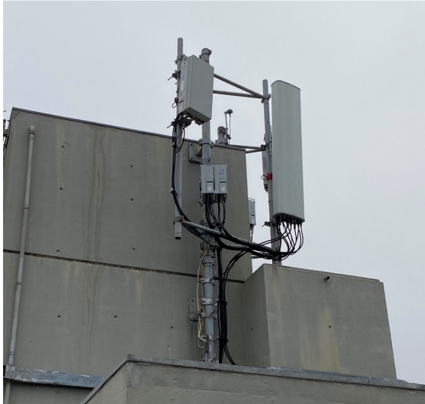
Figure C.3. Point of view from the lower terrace to sector 1 of BS1.
