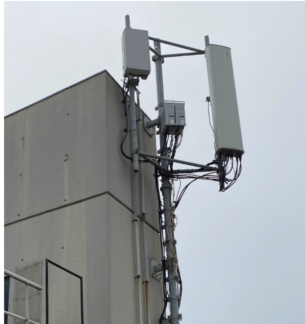
Figure C.6. Point of view from the lower terrace to sector 2 of BS1
